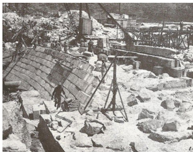
Fig. 2: General view of the wall under construction (City of Cape Town 1921)
